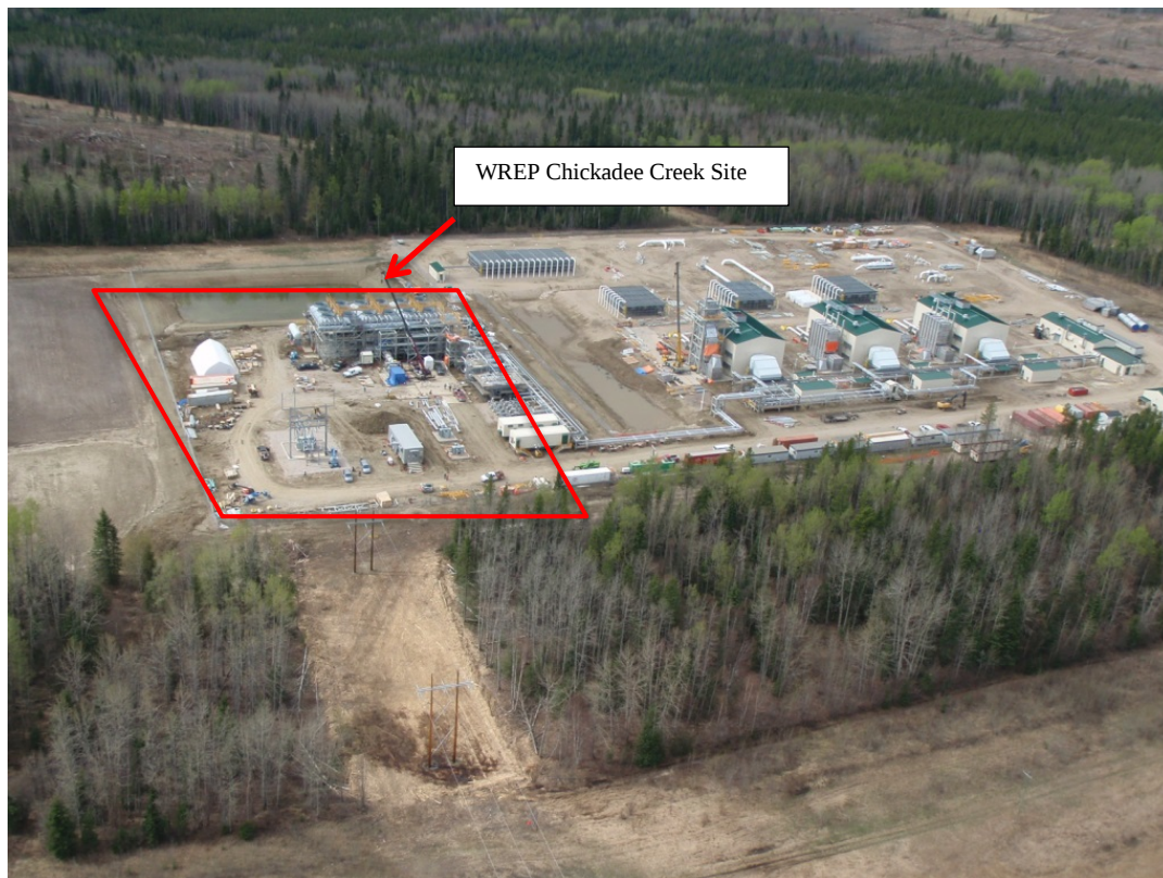
Figure 4: Chickadee Creek and Windfall Compressor Site Construction
