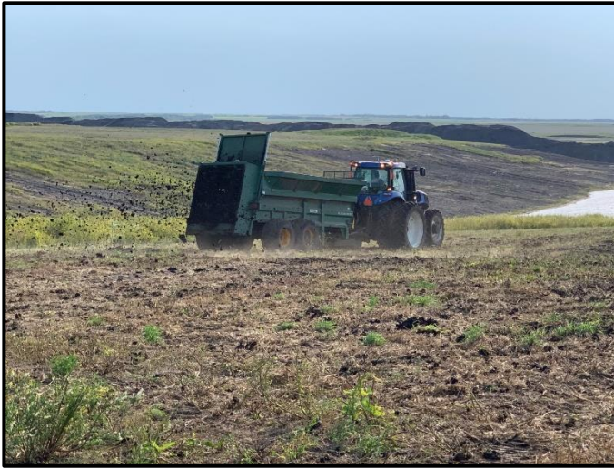
Photograph 2: Biosolids were applied directly to subsoil as an alternative to topsoil placement. The organic matter and nutrients from the biosolids support vegetation growth, allowing the subsoil to develop into topsoil. (June 2020)
